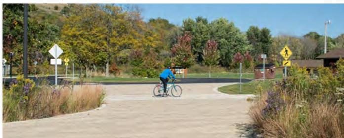
Permeable pavement & bioretention bump-outs
