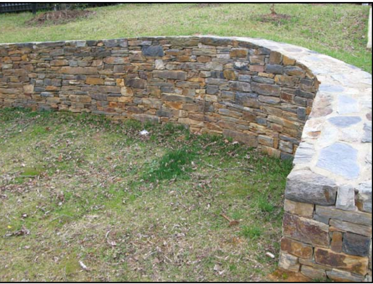
Precedent Example of stone work Duke stone coursing and inset hidden joints with fully mortared cap.
