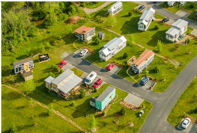
Bungalow Court (top left) Pocket Neighborhood (top right) Tiny Home Neighborhood (bottom left)
