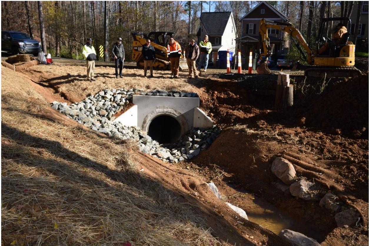
**Project Description:** This project involved replacing an old and undersized culvert on the 400 block of Broad Street.
