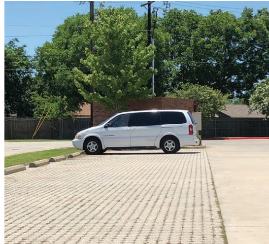
Pervious pavement in parking stalls
