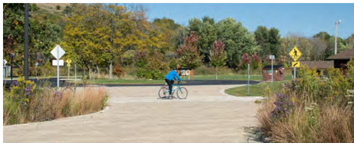
Permeable pavement & bioretention bump-outs
