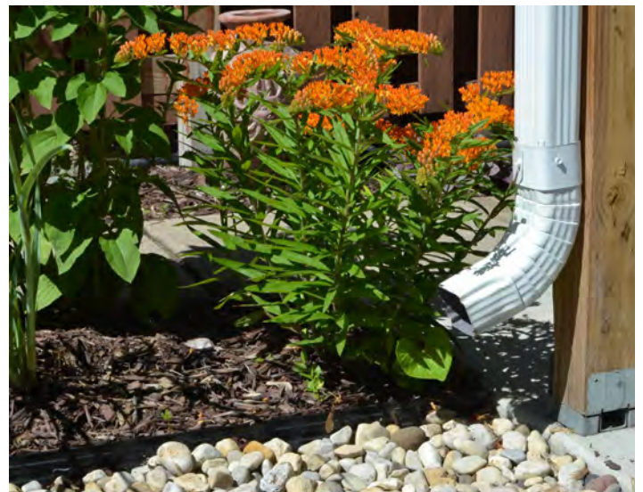
Impervious removal and disconnection
