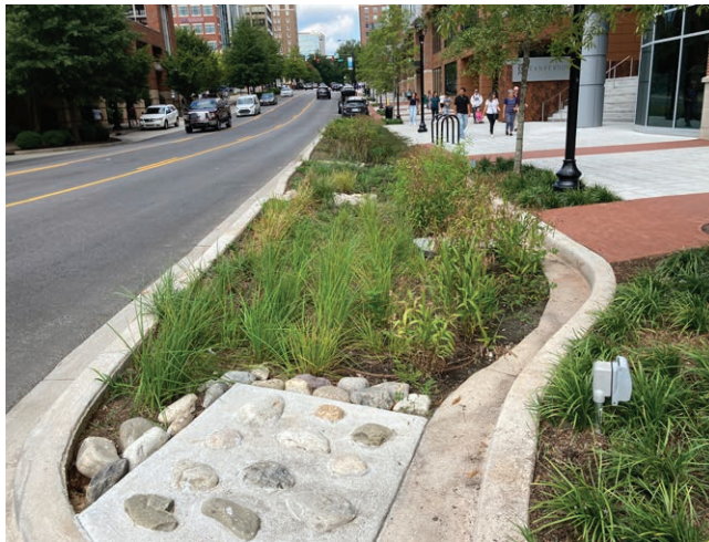
Pervious strips capture and slow runoff
