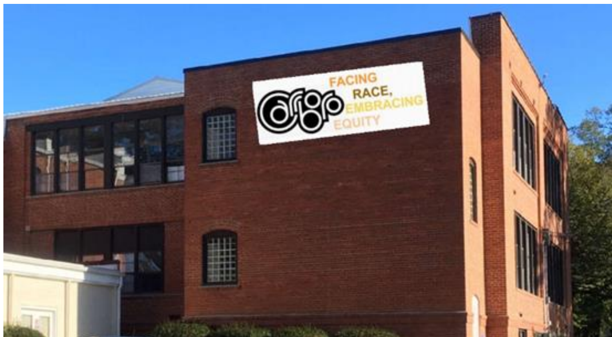
Stair tower south view
