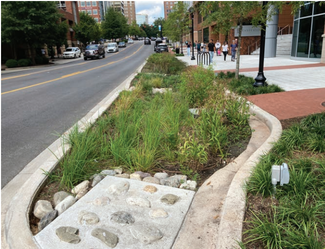
Pervious strips capture and slow runoff
