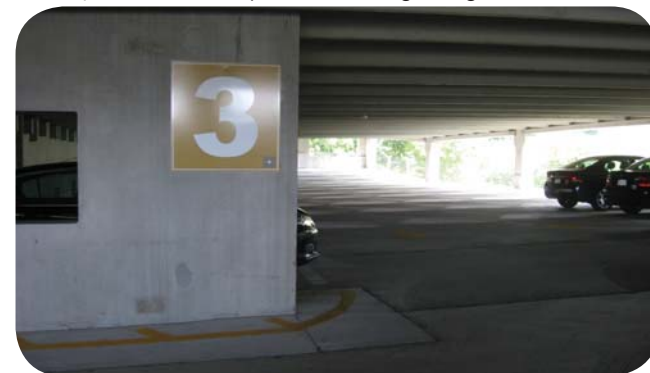
Photo 1 | Level 3 of Hampton Inn Parking Garage
