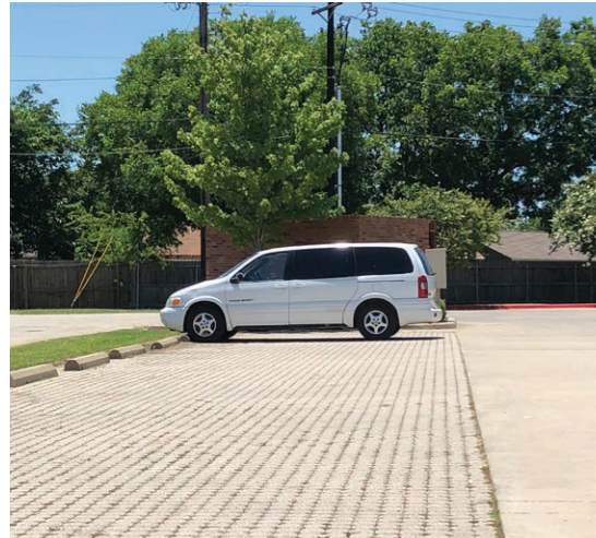
Pervious pavement in parking stalls
