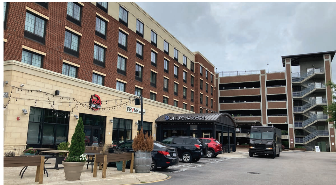
Existing parking garage in downtown
