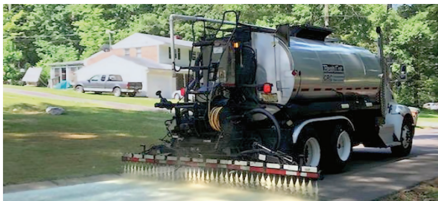
PlusTi A.R.A.-1 Ti® asphalt rejuvenator/sealer application
