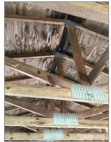
Picnic Shelter Roof
