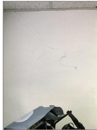
Second Floor - Plaster Walls
