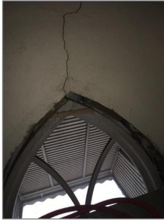
Attic - Exterior Wall
