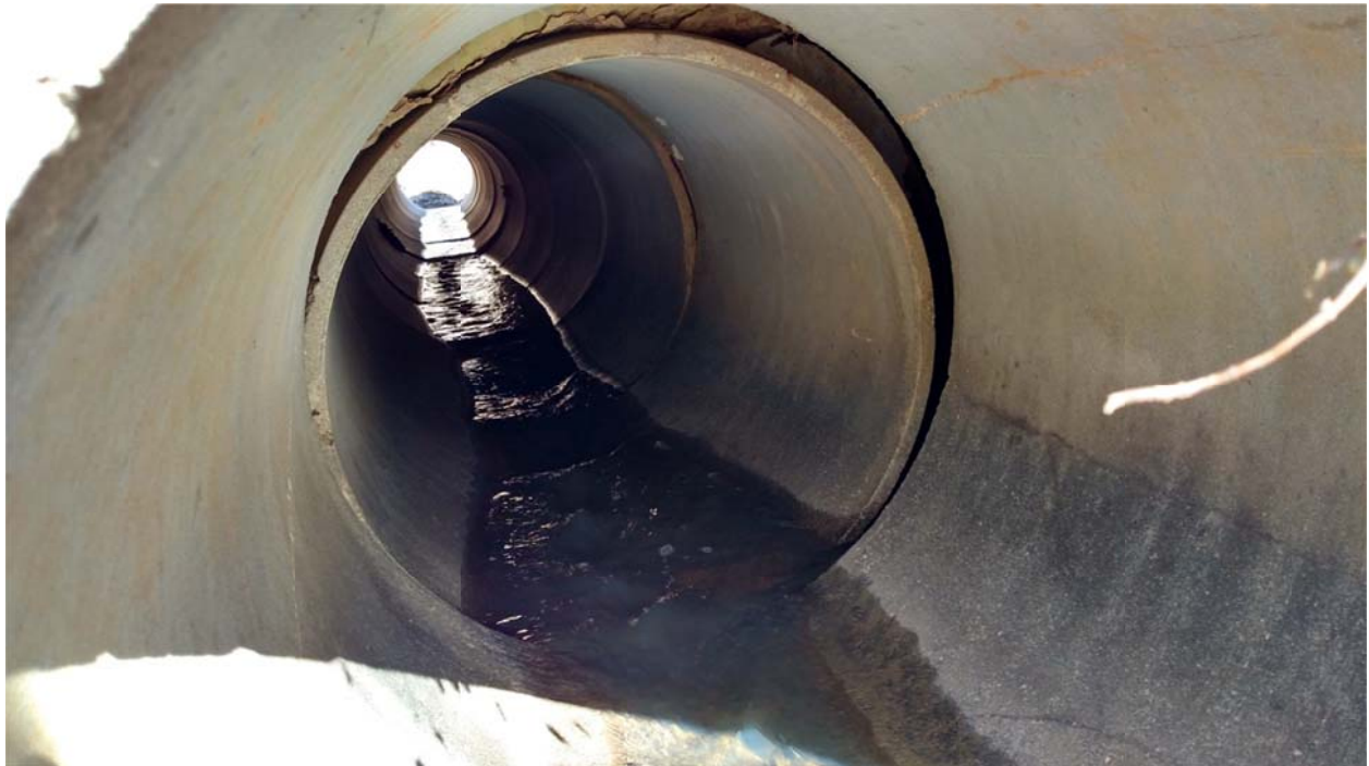
Looking inside 36” Concrete Pipe – Pipe Separation
