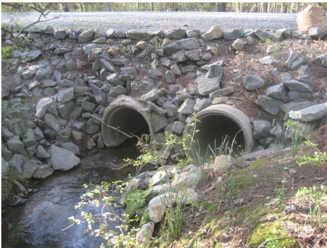
Upstream Face – 2 @ 30” Concrete Pipes
