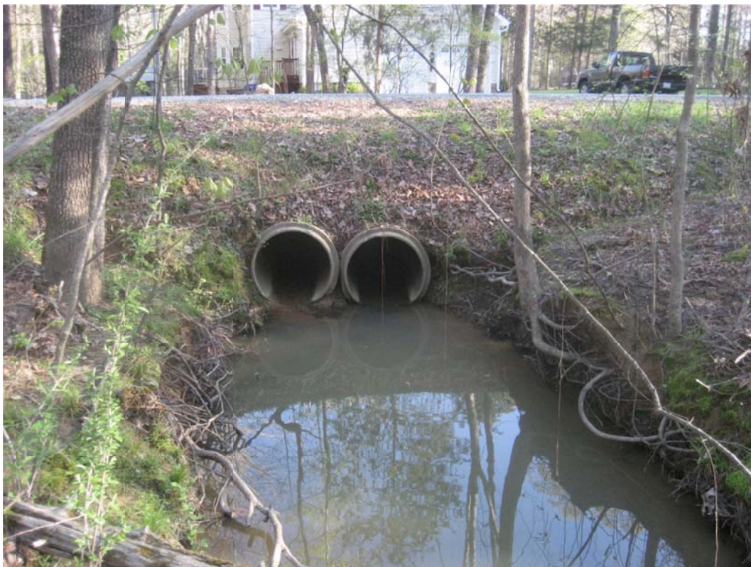
Downstream Face – 2 @ 30” Concrete Pipes
