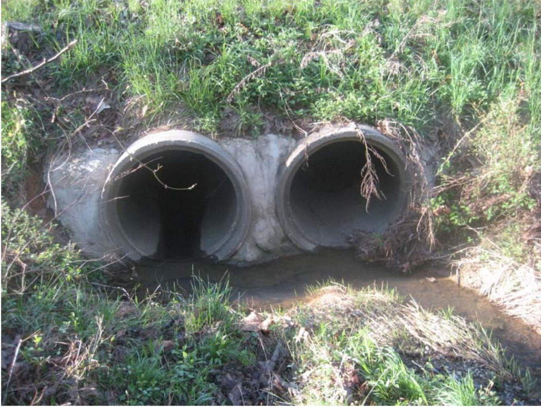
Upstream Face – 2 @ 36” Concrete Pipes
