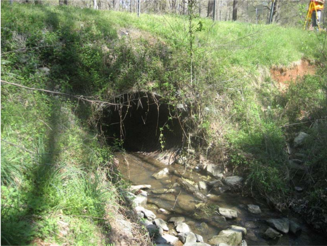
Downstream Face – 1 @ 66" Corrugated Metal Pipe
