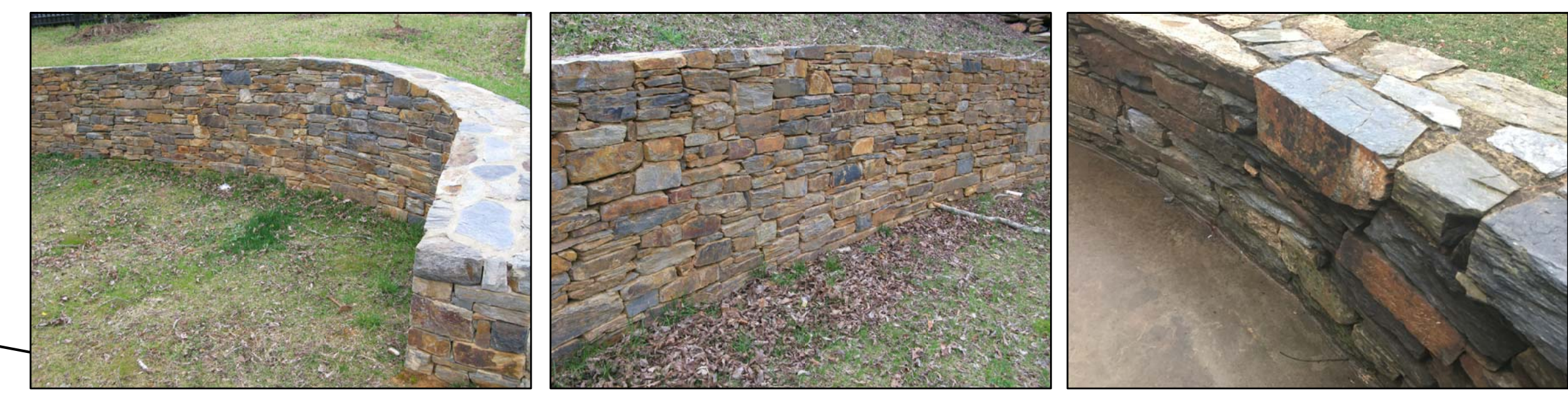
Precedent Example of stone work Duke stone coursing and inset hidden joints with fully mortared cap.
