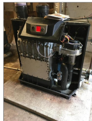
1 st Floor Boiler for HVAC
