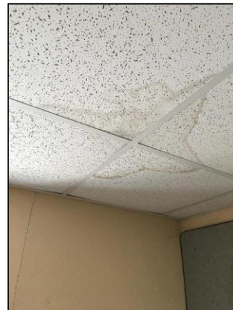
Damaged Ceiling Tiles
