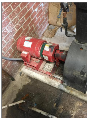
Hot Water Pump for HVAC
