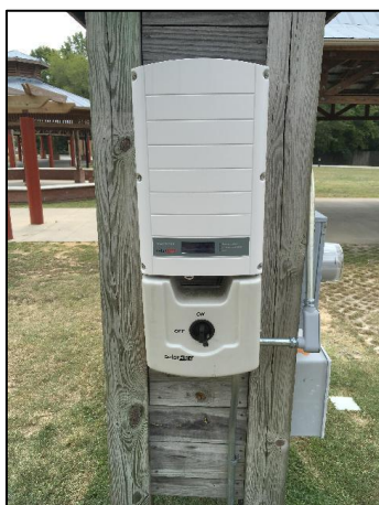
Power Inverter for Solar Panels
