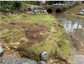
**Project Description:** This project has involved two phases of repairing/restoring a badly eroding stream channel in an extremely high risk situation adjacent to Public Works. The first phase was preliminary engineering; the second is construction/restoration.
