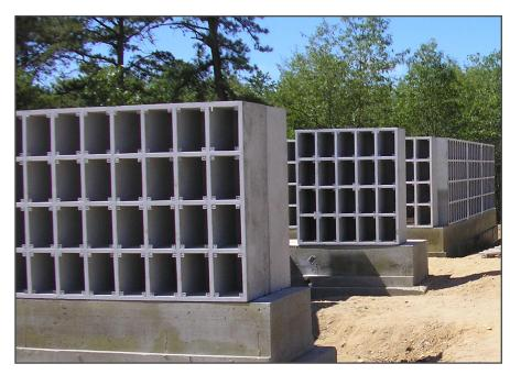
Figure 37 Columbaria under construction, with pre-cast concrete niches visible. (CVDA)
