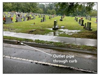
Figure 20 On Fidelity Street, tree roots create a ponding issue that could be resolved by connecting an inlet to the existing drain pipe. (CVDA)
