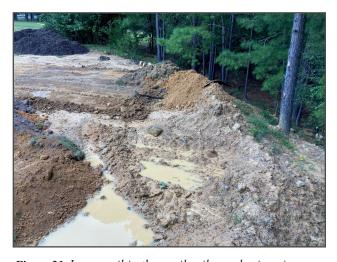
Figure 21 Loose soil in the spoils pile erodes in rain storms. This area was graded and cleaned up in November 2020. (CVDA)
