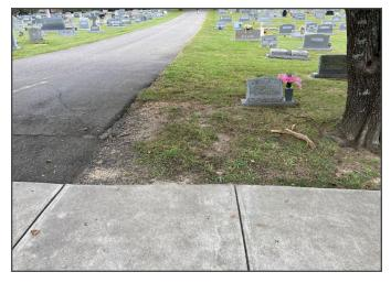
Figure 11 Erosion and root damage are visible along the south side of the driveway apron at Davie Road, in Section 2, looking east. (CVDA)
