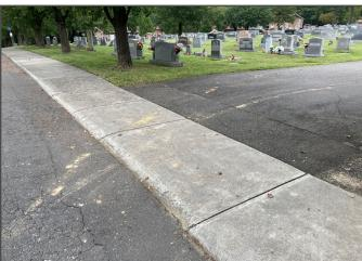
Figure 10 The entrance to the cemetery from Davie Road, between Sections 1 and 2, showing recent asphalt patching, and the sidewalk and driveway apron. The driveway apron is not separated from the adjacent sidewalk and does not have curbing. The sidewalks do not continue into the cemetery. (CVDA)
