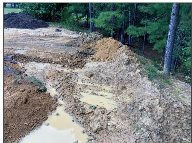
Figure 21 Loose soil in the spoils pile erodes in rain storms. This area was graded and cleaned up in November 2020. (CVDA)
