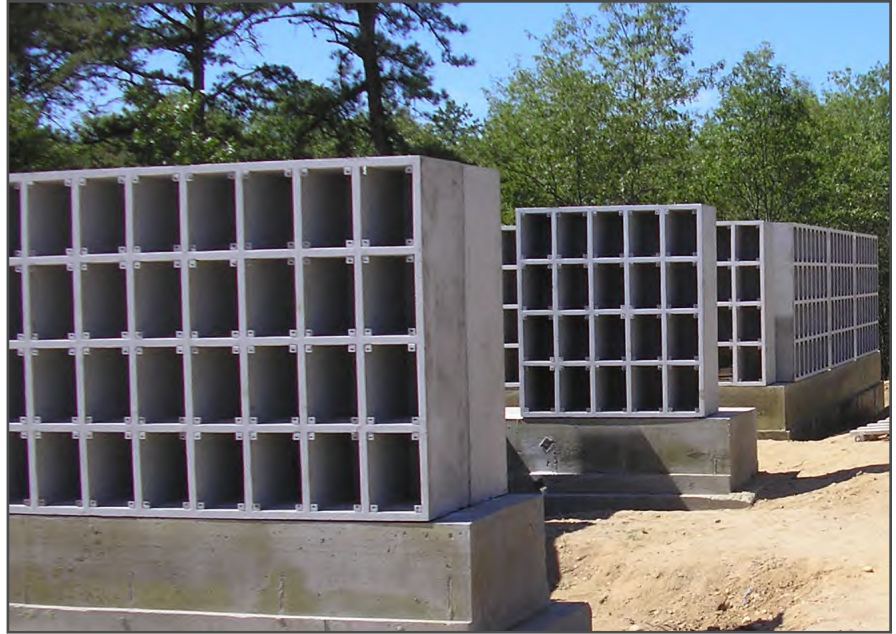
Figure 37 Columbaria under construction, with pre-cast concrete niches visible. (CVDA)
