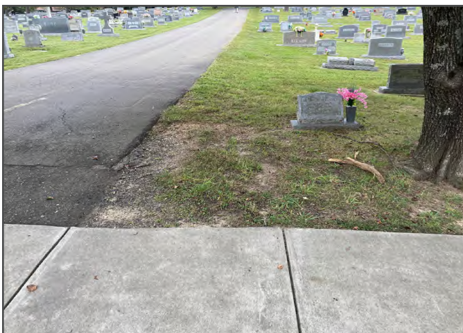
Figure 11 Erosion and root damage are visible along the south side of the driveway apron at Davie Road, in Section 2, looking east. (CVDA)
