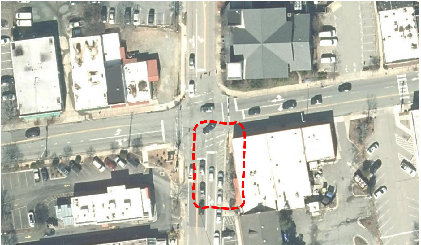
Loading zone prior to resurfacing
