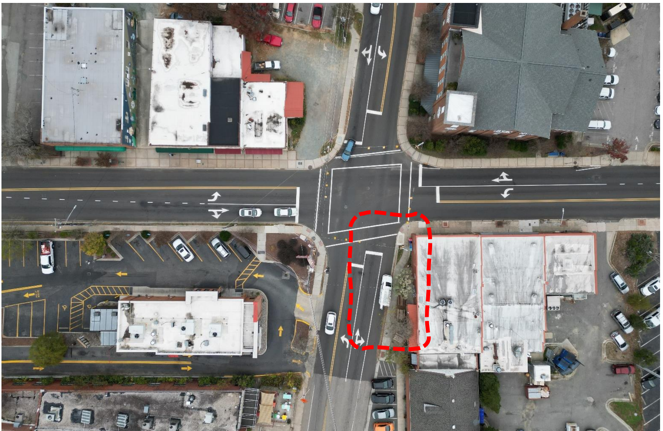
Loading zone removed after resurfacing
