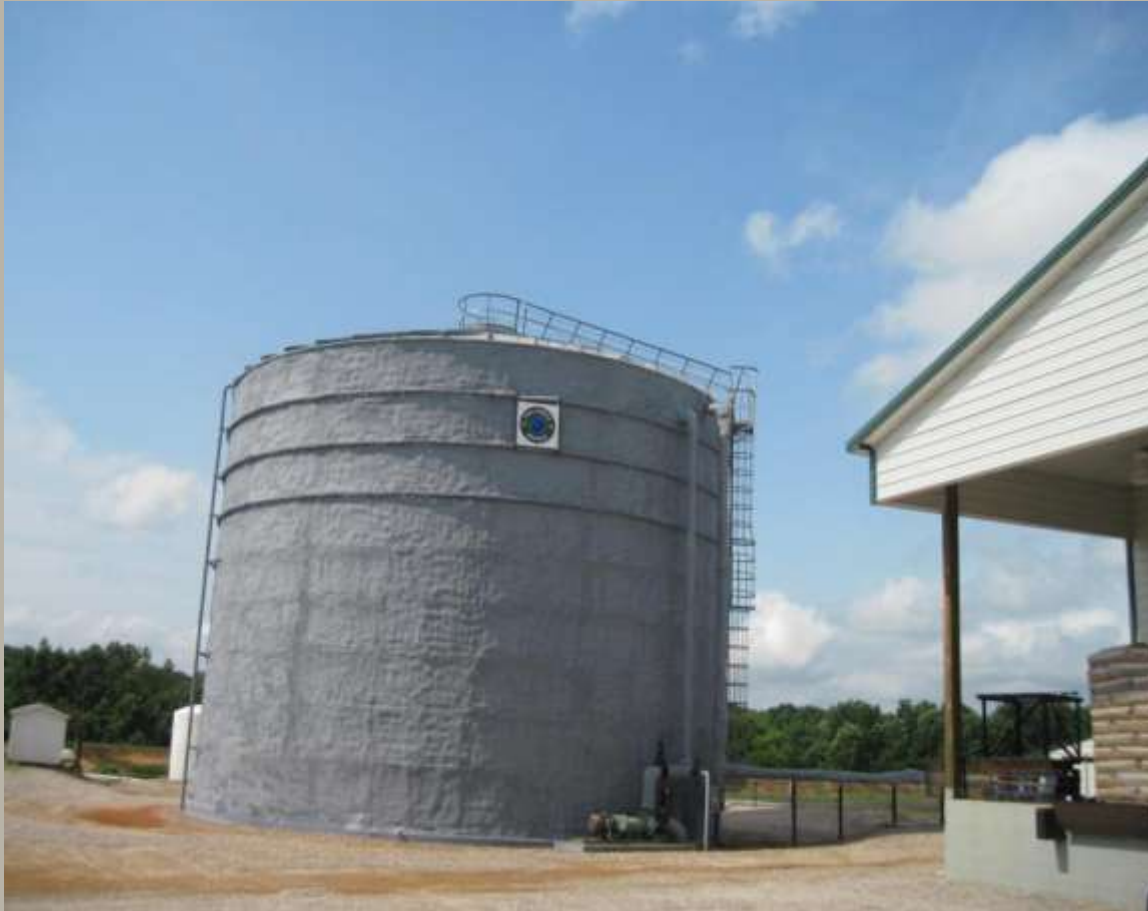
Anaerobic Digester Accepting Food Waste
