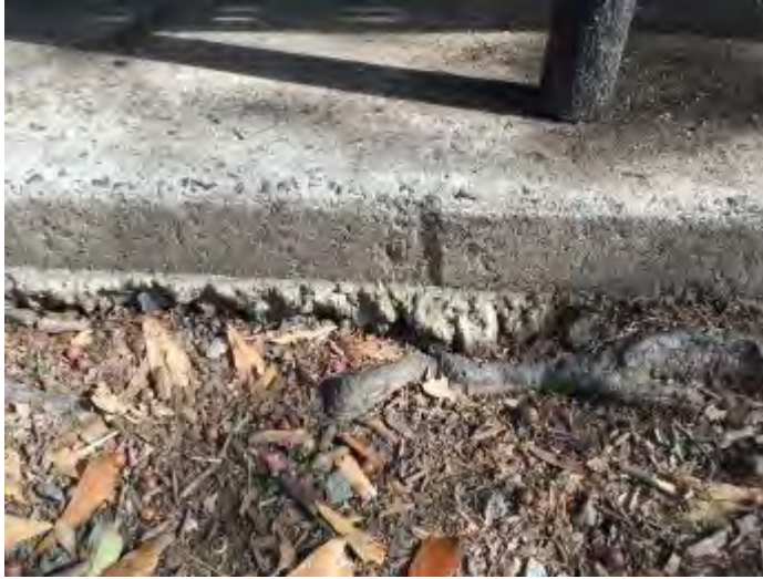
Photo - Edge of sidewalk at Weaver St. Market. Note erosion and exposure of un-formed concrete. The Yard was once flush with the sidewalk.
