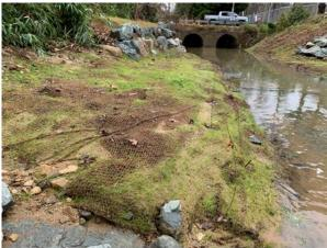
**Project Description:** This project has involved two phases of repairing/restoring a badly eroding stream channel in an extremely high risk situation adjacent to Public Works. The first phase was preliminary engineering; the second is construction/restoration.
