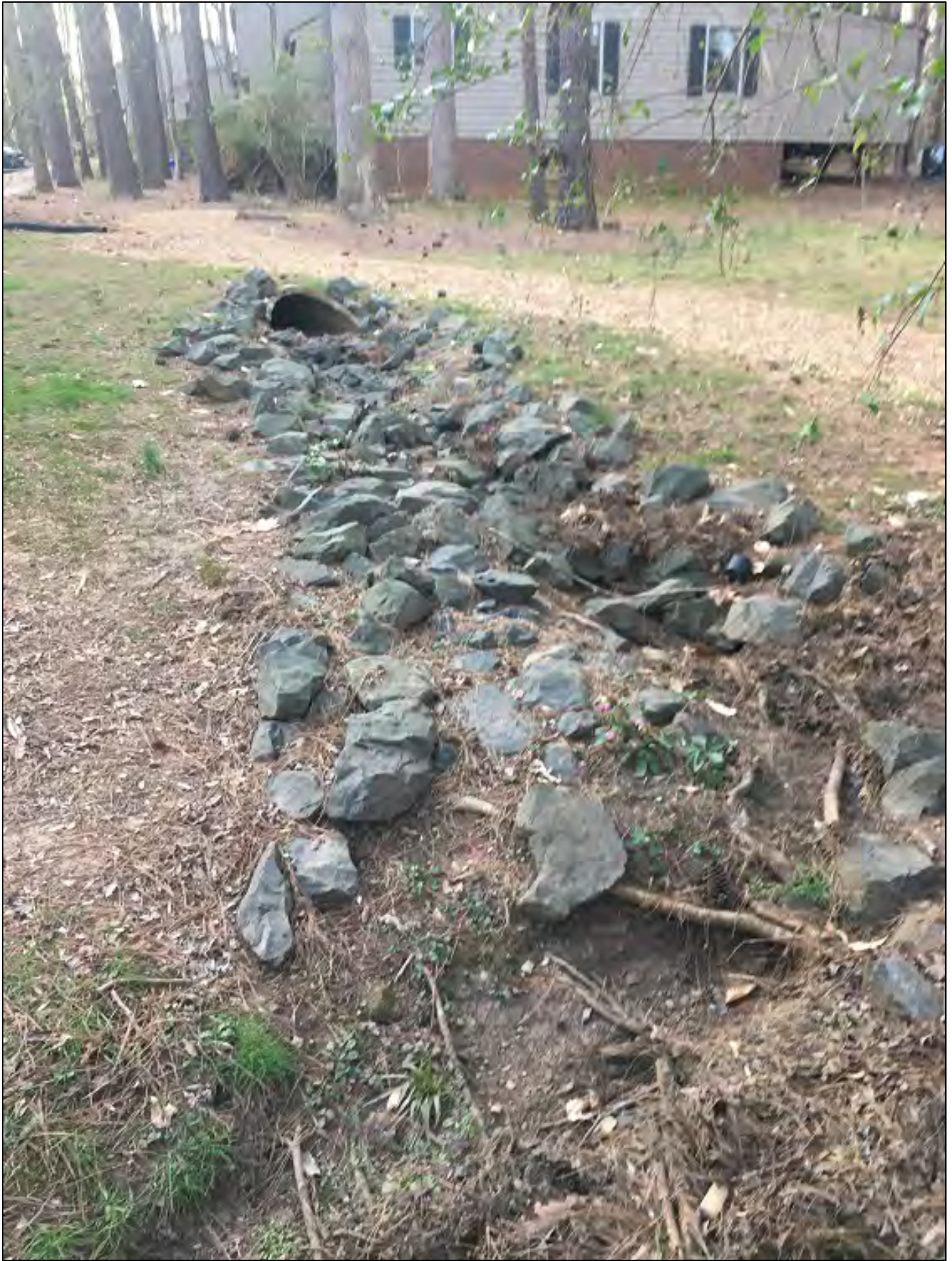
PICTURE 4 – BOULDER POOLS TO BE LOCATED AT FOREST COURT PIPE OUTFALL
