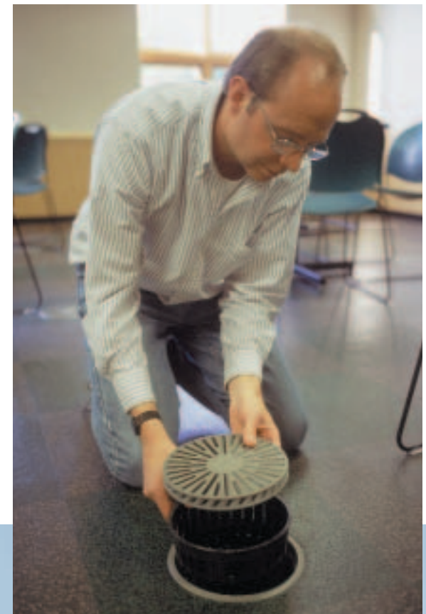
Checking air flow in a displacement ventilation system diffuser. Dirty or clogged air filters are a common commissioning finding. Not only do dirty filters reduce air handler efficiency, they also can affect occupant comfort and health.
