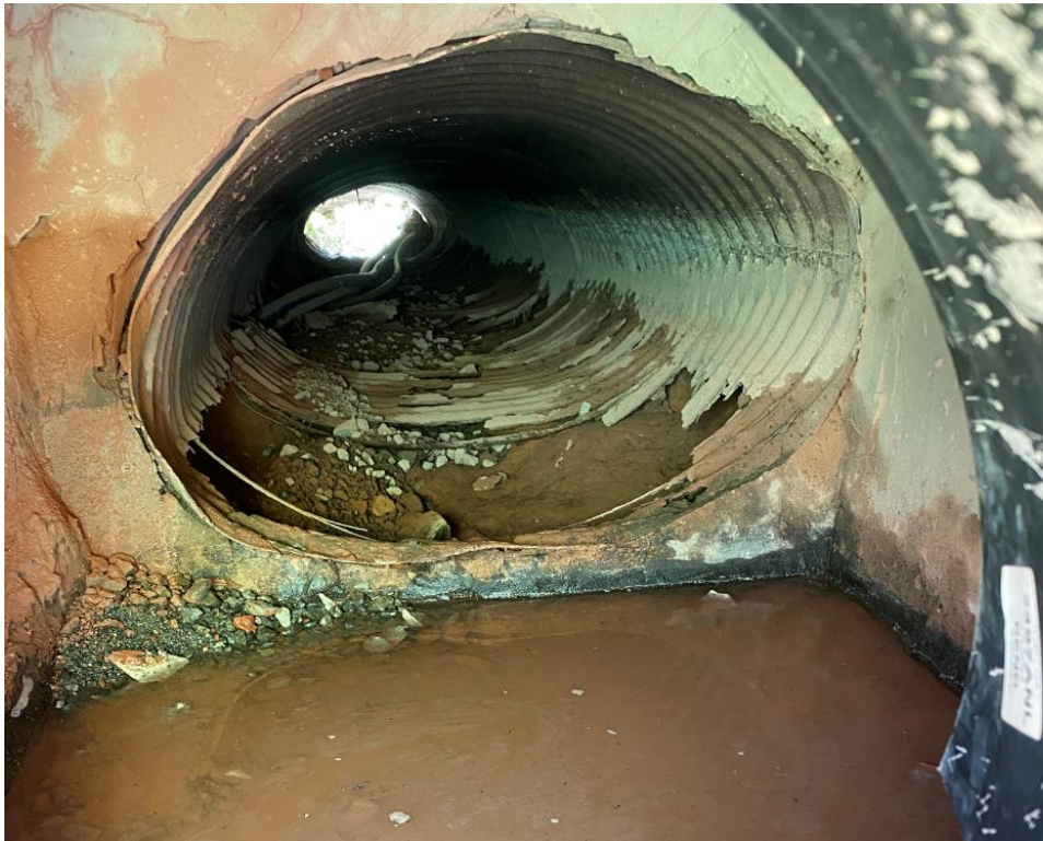
Exhibit 1: Existing Carr St. Culvert (Previous design included reusing this infrastructure)
