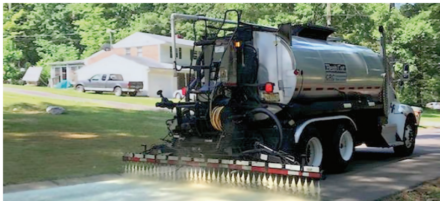
PlusTi A.R.A.-1 Ti® asphalt rejuvenator/sealer application
