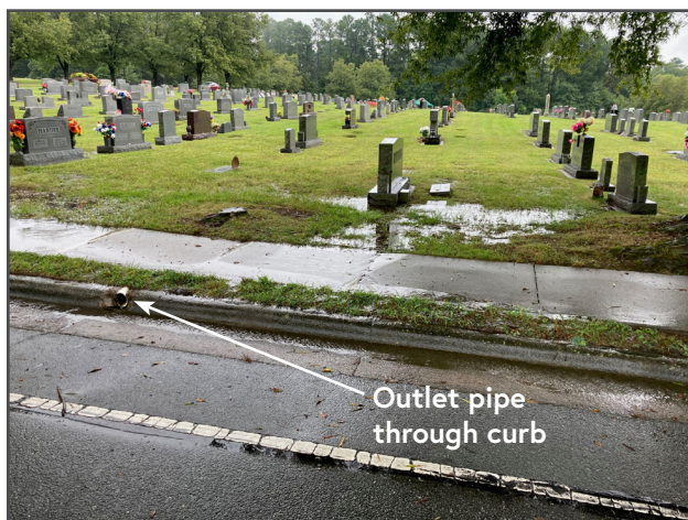
Figure 20 On Fidelity Street, tree roots create a ponding issue that could be resolved by connecting an inlet to the existing drain pipe. (CVDA)
