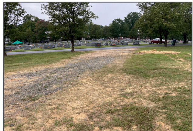
Figure 26 Contractor damage to the turf in Zone 4 and resulting erosion. (CVDA)
