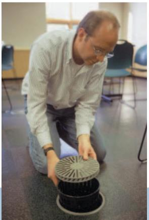
Checking air flow in a displacement ventilation system diffuser. Dirty or clogged air filters are a common commissioning finding. Not only do dirty filters reduce air handler efficiency, they also can affect occupant comfort and health.
