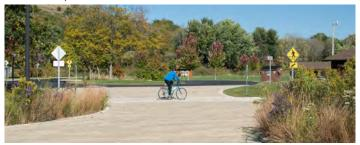
Permeable pavement & bioretention bump-outs
