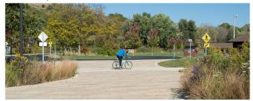
Permeable pavement & bioretention bump-outs
