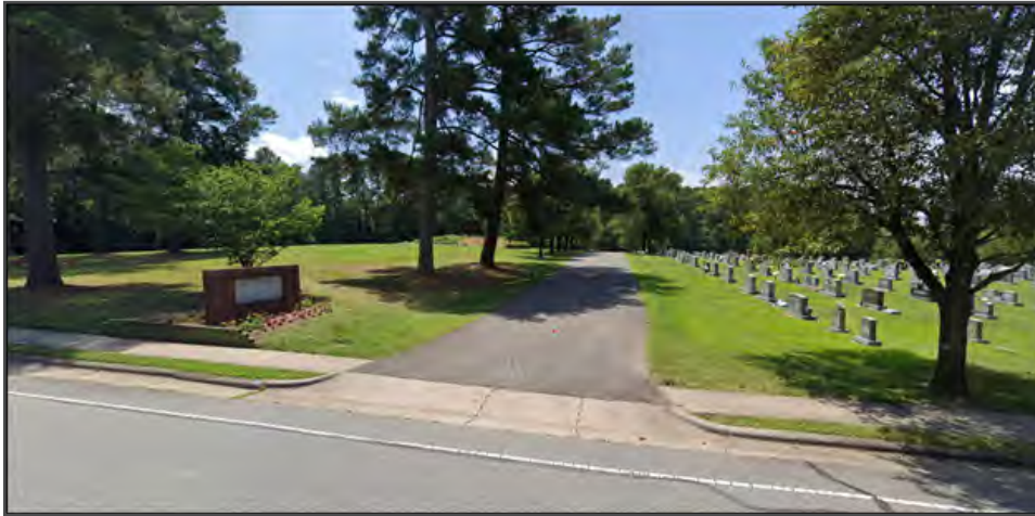
Figure 10 The entrance to the cemetery from Davie Road, between Sections 1 and 2, showing recent asphalt patching, and the sidewalk and driveway apron. The driveway apron is not separated from the adjacent sidewalk and does not have curbing. The sidewalks do not continue into the cemetery. (CVDA)
