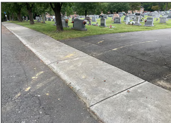
Figure 10 The entrance to the cemetery from Davie Road, between Sections 1 and 2, showing recent asphalt patching, and the sidewalk and driveway apron. The driveway apron is not separated from the adjacent sidewalk and does not have curbing. The sidewalks do not continue into the cemetery. (CVDA)
