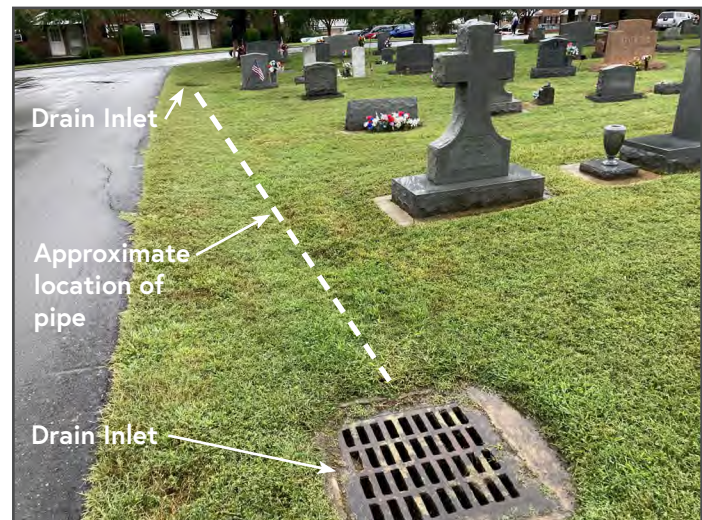
Figure 19 Interconnected drain inlets leading to the stormwater system at Davie Road. (CVDA)
